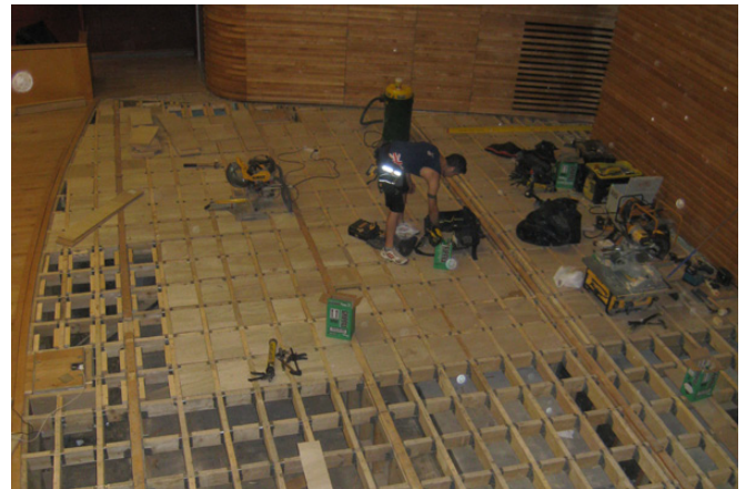
Hall floor being rebuilt — Photo Credit: Brian Fifield
